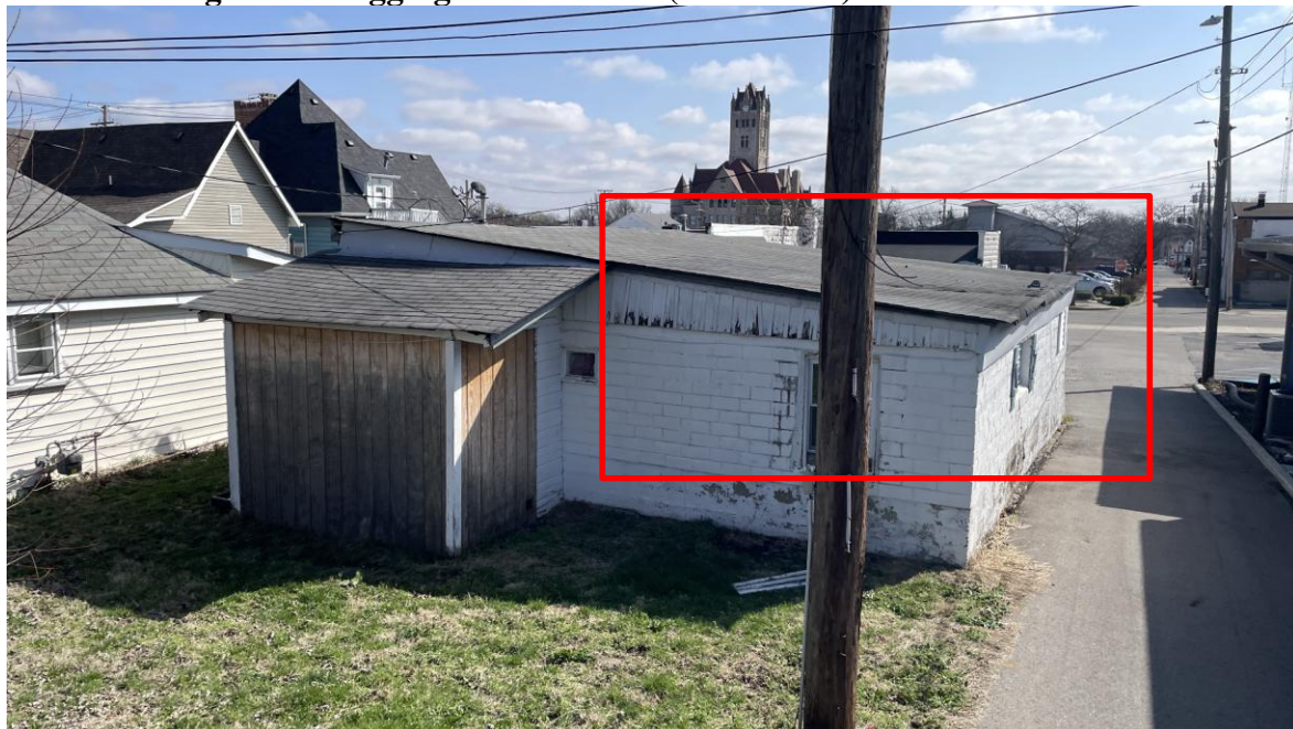
Back Building's Roof sagging in the middle (like a bowl)
